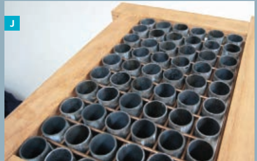
copper rods) can be substituted for cable ties. Fig. J: After the wooden frame is expanded, it can be retightened around the wider-spaced conduits.
