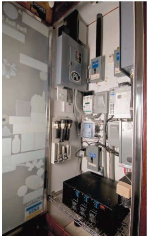
ABOVE: AGM battery bank stores solar power for the studio, while a banjo provides inspiration to visiting cowboy poets. RIGHT: Power center contains all the equipment needed for off-grid electrical generation.
