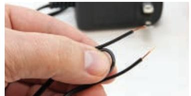
**3b.** Solder a piece of wire to each end of the cut wire, and seal both connections with some heat-shrink tubing.
