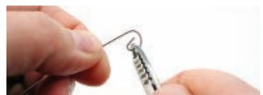
**2c.** To electrically insulate the guitar wire from the wall anchor, cut two ½"-long pieces of ⅛" heat-shrink tubing, then slip and shrink them one by one over the wire at the lug end.
